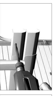
Drill the marked holes  $\varnothing$ 8.5 mm.
